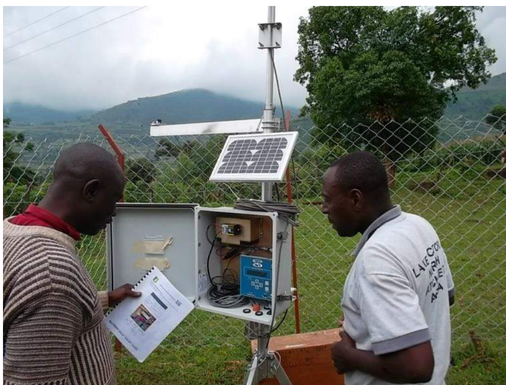
Figure 4: Technical Officers from LVNCA taking readings from an automatic weather station at Bumbe installed by the SMM Project (SMM, 2011).
